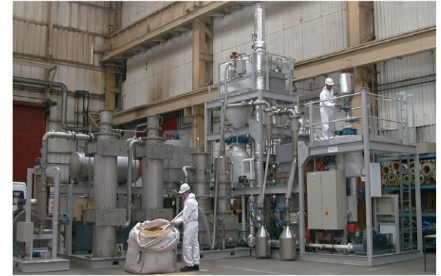
250 kg/h pilot plant at Wellman, UK
