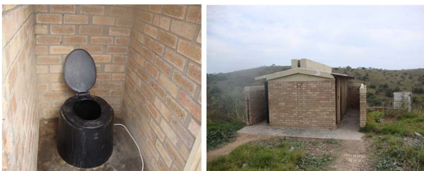
Figure 2. Pit latrine system that was installed in Chintsa Primary School, Eastern Cape, South Africa that will be soon to be replaced by Integrated Biogas and Algal biogas system.
